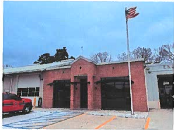
Station 31 Exterior Remodel
